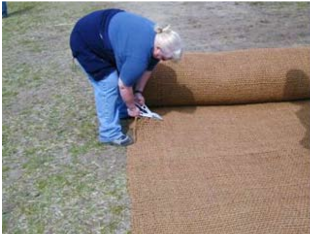
Figure TS14I-38 Cutting coir fabric ( Photo courtesy of Sonia Jacobson, NRCS )
