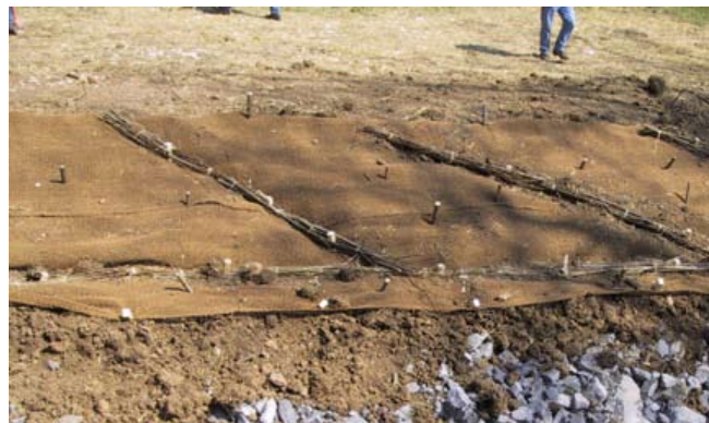
Figure TS14I-24 Fascines installed at an angle over a riprap toe
