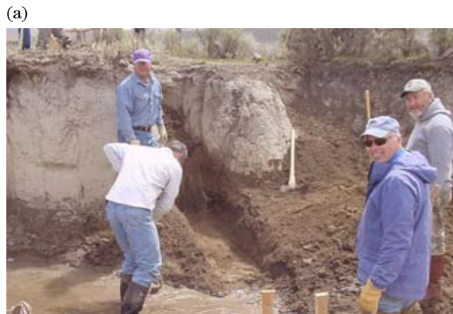
Figure TS14I-13 Brush spur being installed
