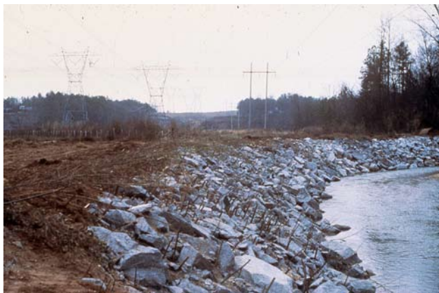
Figure TS14I-25 (a) Completed installation of joint planting; (b) Early in first growing season ( Photo courtesy of Robbin B. Sotir & Associates, Inc. )
