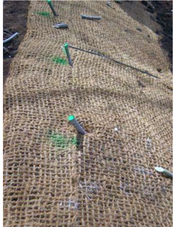
Figure TS14I-39 Live cuttings installed in fabric
