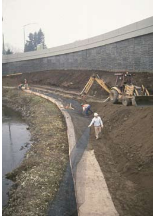
Figure TS14I-31 Geogrid wrapping of soil lift ( Photo courtesy of Robbin B. Sotir & Associates, Inc. )
