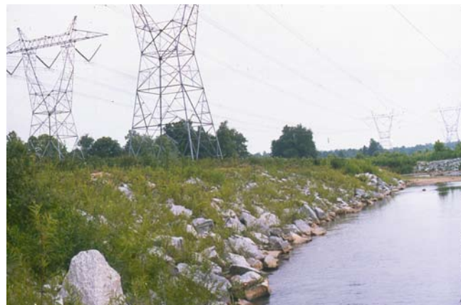
Figure TS14I-25 (a) Completed installation of joint planting; (b) Early in first growing season ( Photo courtesy of Robbin B. Sotir & Associates, Inc. )
