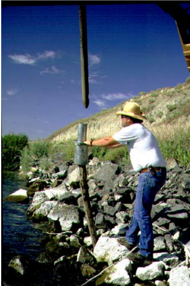
Figure TS14I-23 Installation of dormant posts with stinger
