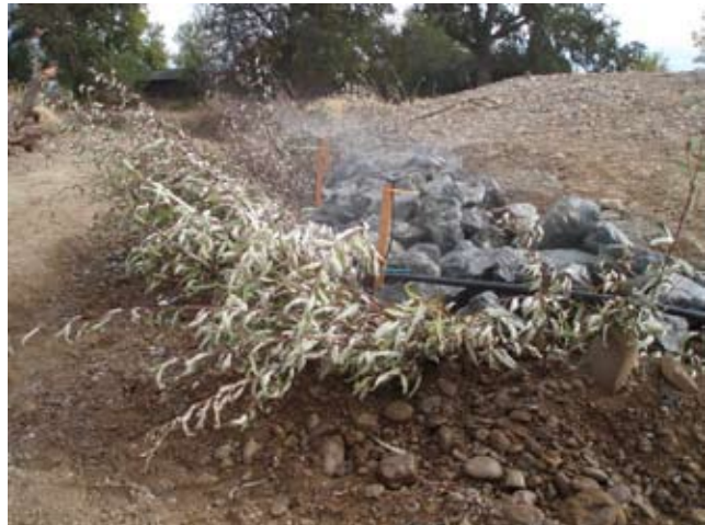
Figure TS14I-16 Live siltation construction or live brush sills with rock
