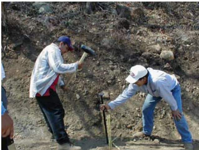
Figure TS14I-21 Iron punch bar being used to create pilot hole
