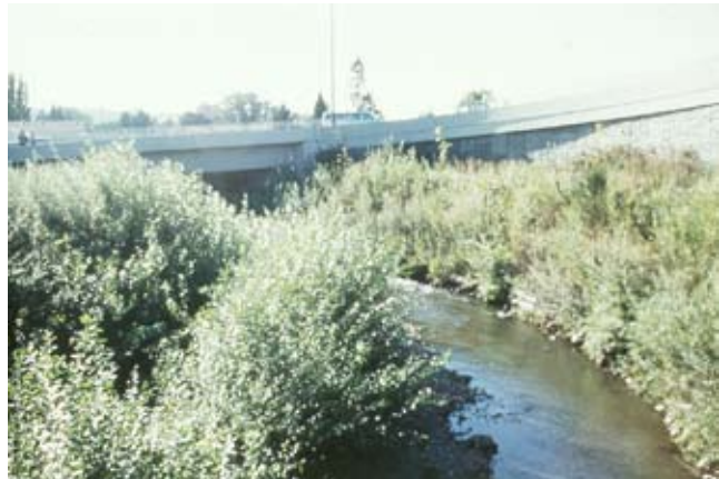
Figure TS14I-33 VRSS development after 4 years ( Photo courtesy of Robbin B. Sotir & Associates, Inc. )
