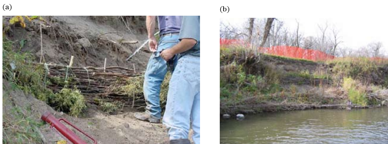
Figure TS14I-34 (a) Wattle fence immediately after construction; (b) 1 year later
